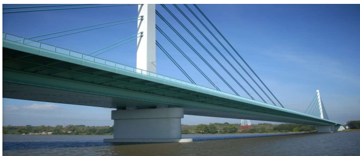
Fig. 1. View of a bridge with suspended system in Płock
